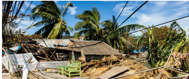
Wooden buildings completely destroyed by the passage of a tropical cyclone. Source: Adobe Stock
